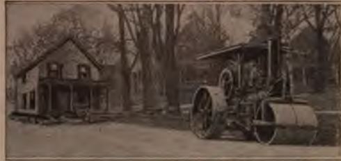
A Small House being Dragged a Quarter of a Mile through the Streets of a Populous Town by a Steam Roller
